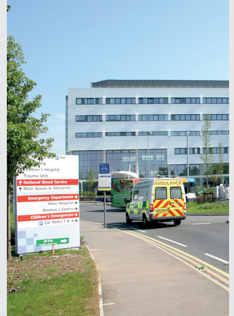
West Wing of the John Radcliffe Hospital
